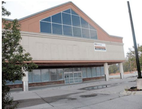
A&P has stopped paying rent on nearly all of its local long-term leases, including for this former Farmer Jack store on 7 Mile in Livonia.
